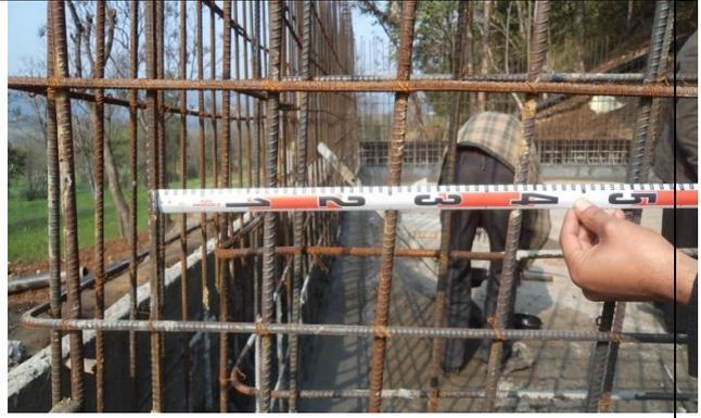
**D-1, D-3 Inspection of R-bars spacing before placing formwork**
