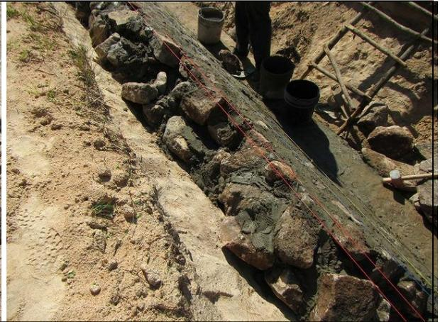
**Walling based on "Good practice (well mixing of Mortar then Stone, from Bottom)**
