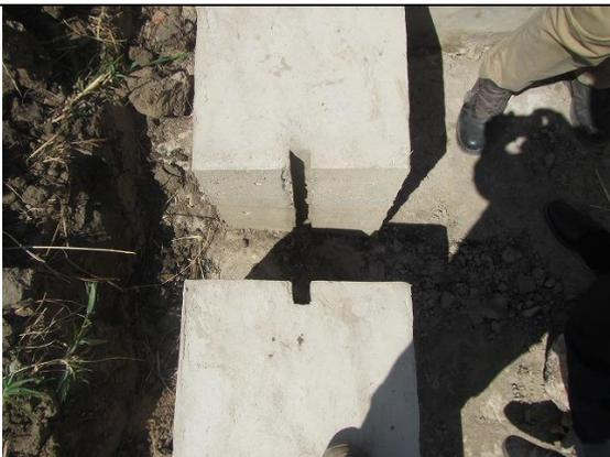
**A pair of Grooves shall be parallel to each other for a smooth operation of gate/ stoplog**
