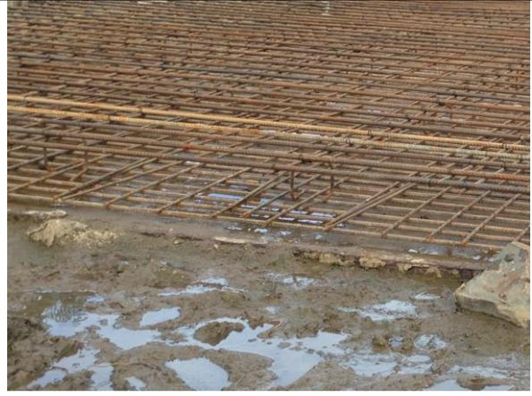
**Blinding Concrete placed first, then R-bar**
