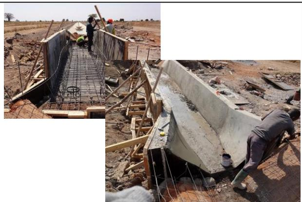
**Transitional section between structure (vertical) and Canal lining (slanting/leaning)**
