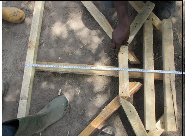
Templates for canal are prepared based on the typical drawing of canal lining
