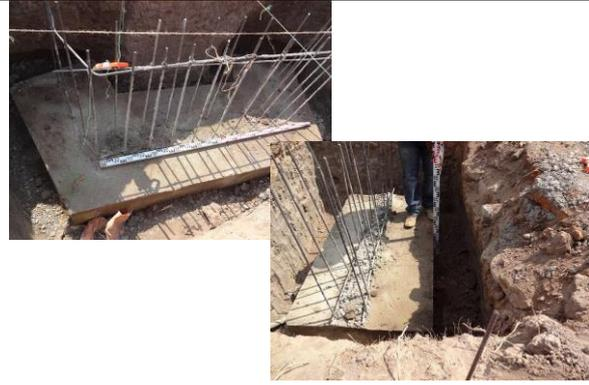
**D-3 Joint Inspection of dimension, EL of base concrete/ footing before walling**
