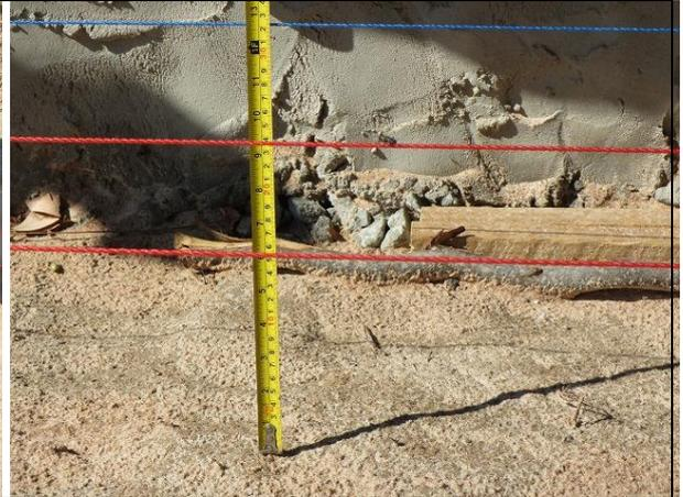
**Inspection of Thickness of the masonry wall (30cm or more, as specified)**
