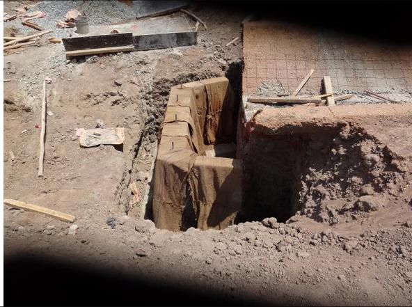
**Curing of structure after placing concrete. Timing and duration is referred to "Curing" See below**
