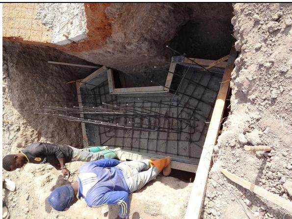
**D-1 Placing of R-bars, setting specified spacing with formwork (footing)**
