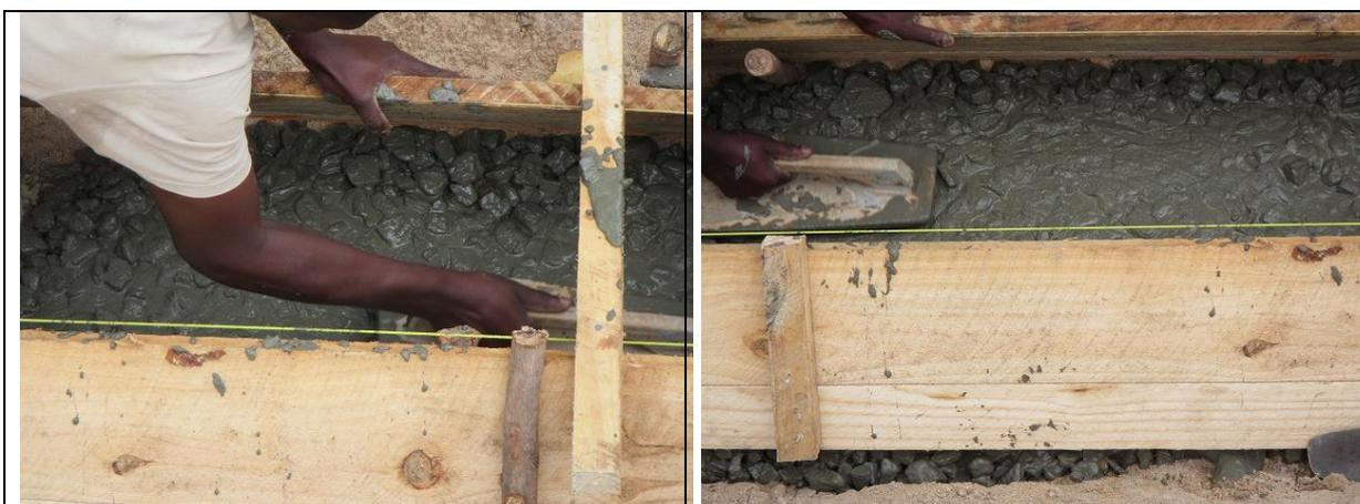
**First concrete layer of plum concrete (5-10 cm)
