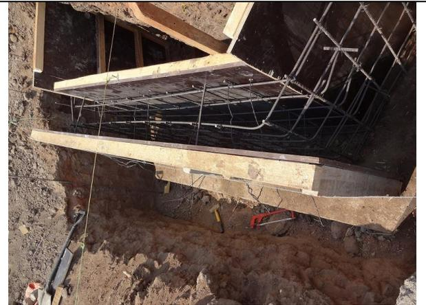
**D-1 Placing of formwork around R-bar for walling**
