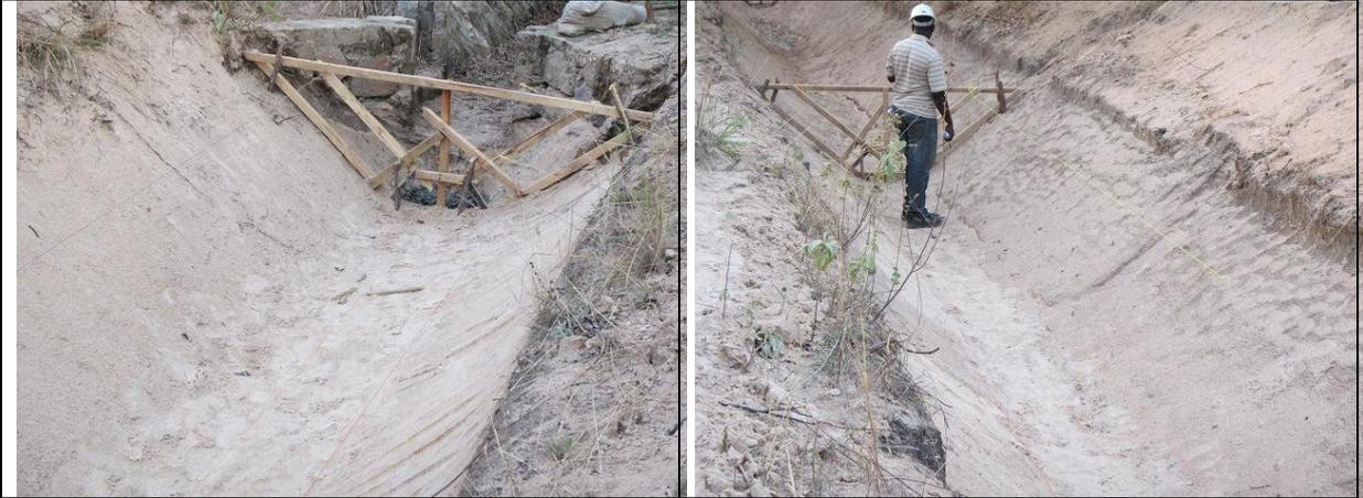
Two consecutive Templates shall be installed at specified chainages and IPs. They have been also set together with 6 - 8 strings, showing lines of lining faces (correct canal bed ELs. And wall lines) and excavation faces (avoid over-excitation)
