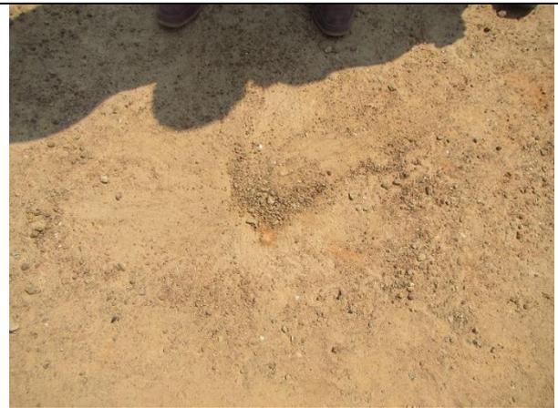
18. (continued) Completion of Restoration of the hole. If it is important to mark clearly for the future works, use pegs (if no traffic), or supplement pegs (to avoid traffic disturbance) (236)
