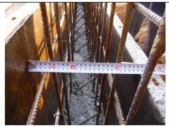
**D-1, D-3 Joint Inspection of spacing between R-bar and formwork before placing concrete wall**
