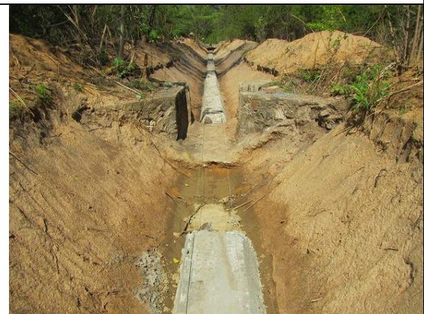
The transition between related structure is also weak point, so that backfill with well compaction is very important
