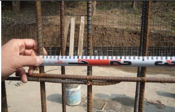
**D-1 Checking of R-bar spacing before placing base concrete/ footing concrete for wall**
