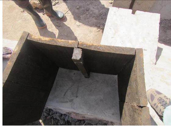
**Preparation of formwork for Grooves**
