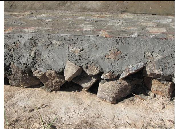
Gap shall be filled by mortar
