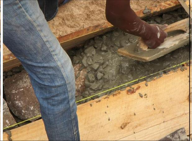
**2<sup>nd</sup> layer of concrete has been placed
