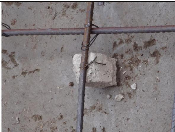
**D-1 Placing of R-bar with spacer block is set on top of blinding concrete**
