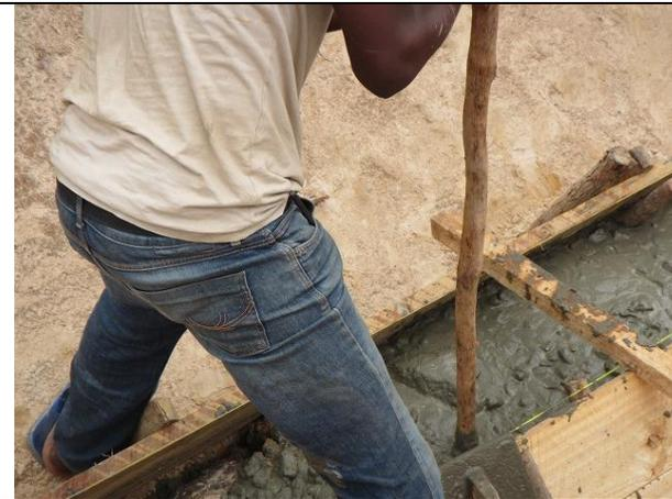
**Hand compaction of 2<sup>nd</sup> layer using rod/
