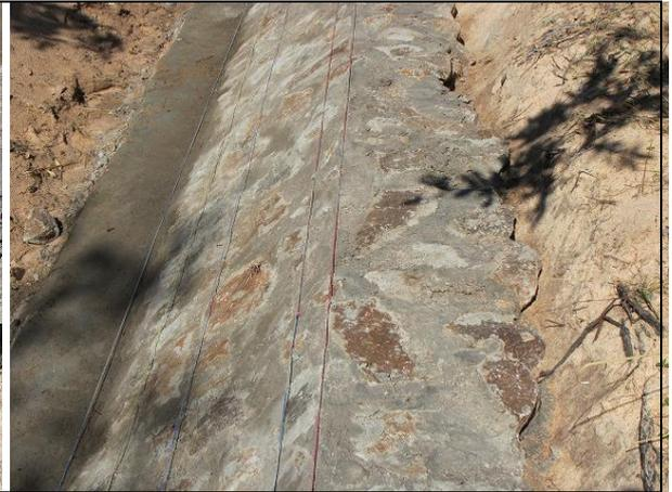
Beam concrete will be placed after filling mortar on the top of the wall
