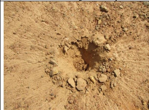
18. After removal of device completely, the hole should be repaired by filling the hole with surrounding soil and pouring water with compaction (236)
