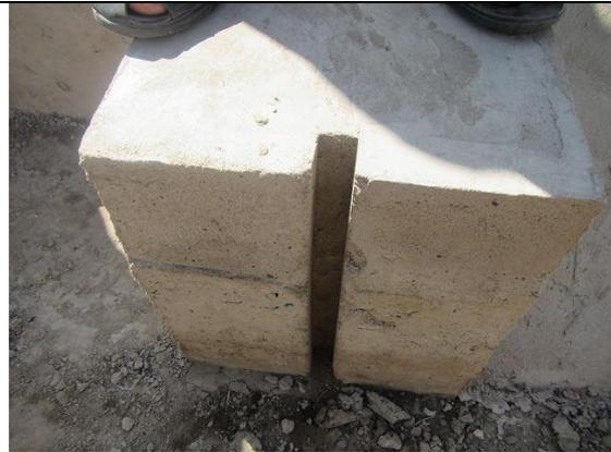
**Wall of division structure with groove (before placing leaning concrete of transition section)**
