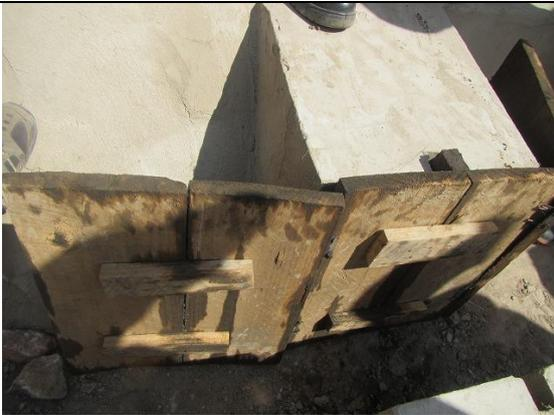
**Concrete Wall with Grooves must be placed before placement of concrete for transition section**
