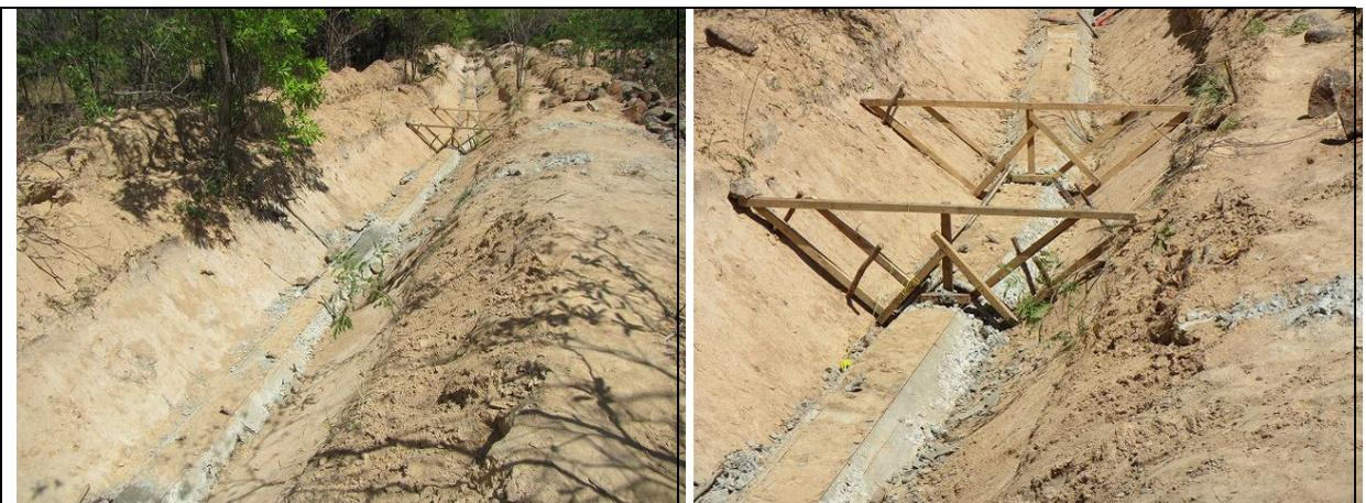
**After hardening (2-3 hours), cured by sand and water for at least 36 hours. Formwork will be removed after 2-3 days**
